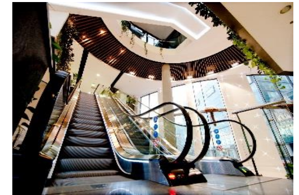
Escalators & Moving Walks
