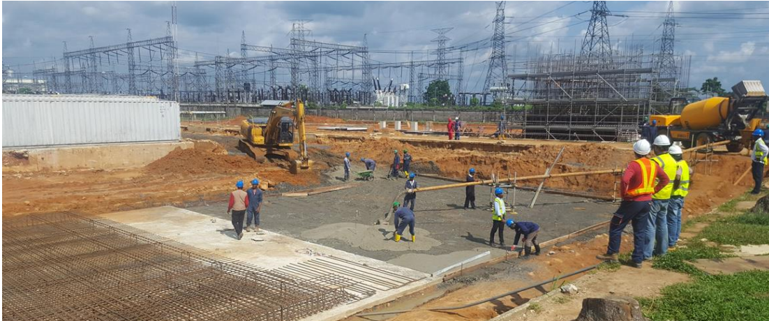
Nigeria – AFAM III (240MW)
